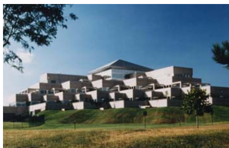
Cedar Rapids Police & Public Safety Facility, Iowa 1997
